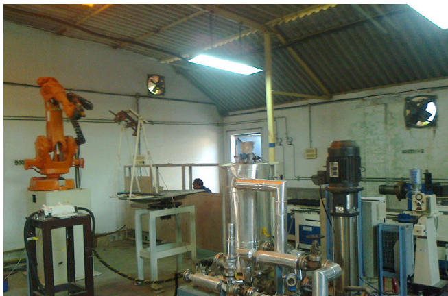
Figure A.2.2.1 Experimental set-up for High Heat Flux testing using Plasma Torch at NFTDC
