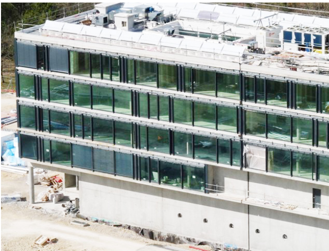
Figure B.2.2.1 : ITER headquarters building
